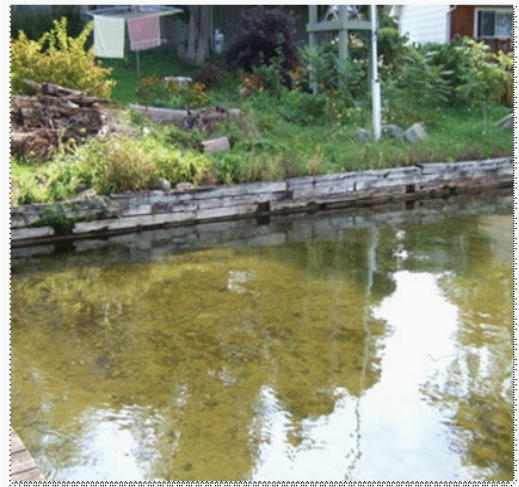
Fig. 2 (Before): Wooden structure holds the soil in place. Photo by Kawartha Conservation
