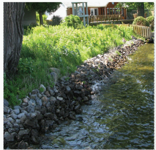
Fig. 3 (After): Sloped rock and natural vegetation provide a healthy and stable shoreline.
