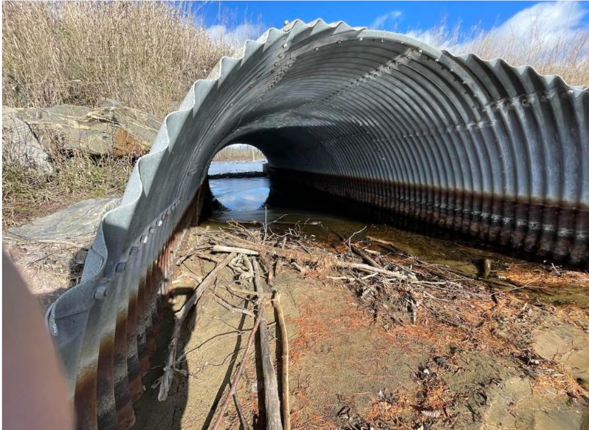
Figure 8 Culvert at Outlet - essentially no flow (GRA)
