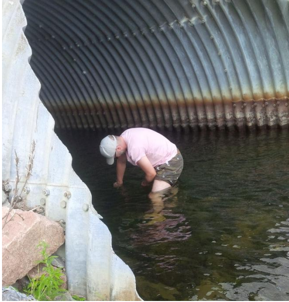
Figure 4 A 5-foot pole being inserted about 4' into the silt. (2019 – West Culvert GRA)
